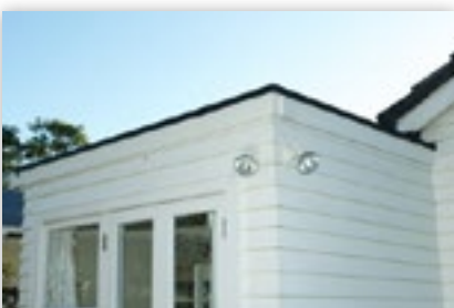
Figure 4: Bitumen membrane skillion roof
