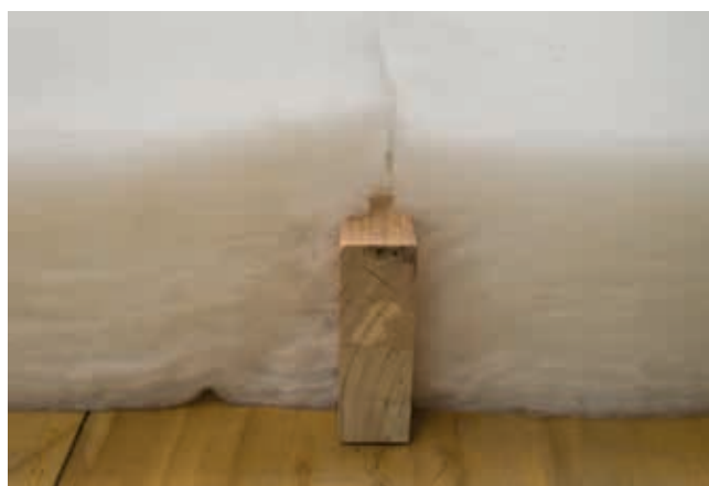
Figure 29 – Friction-fitting insulation over joists
