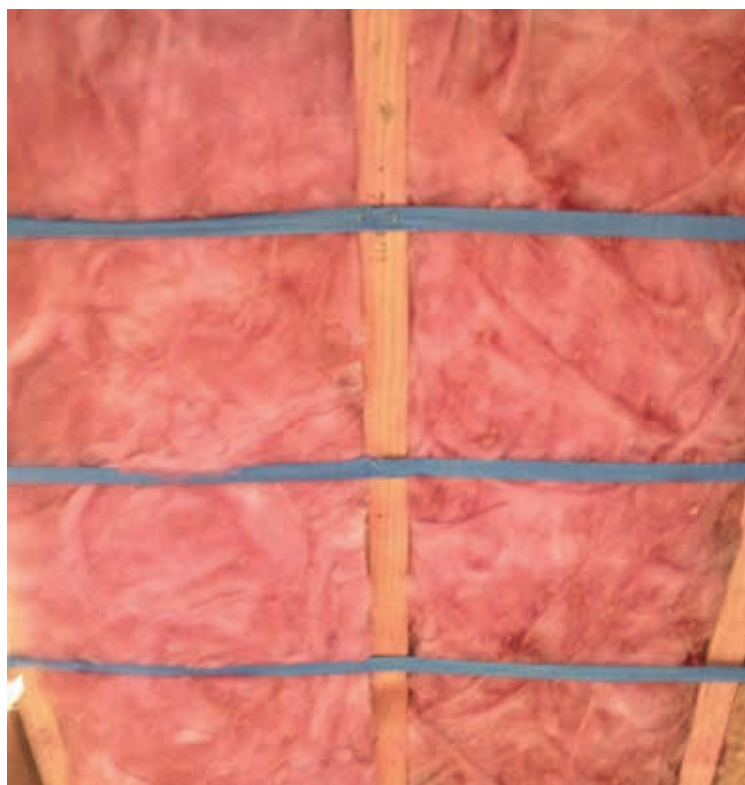
Figure 28 – Blanket in a ceiling secured with strapping
