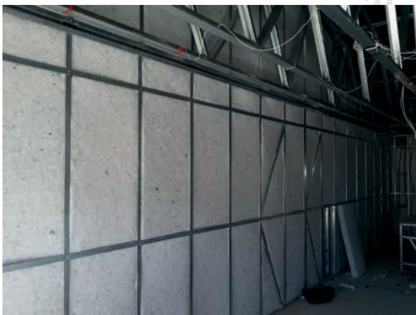
Figure 16 – Insulation fitted into a steel-framed wall
