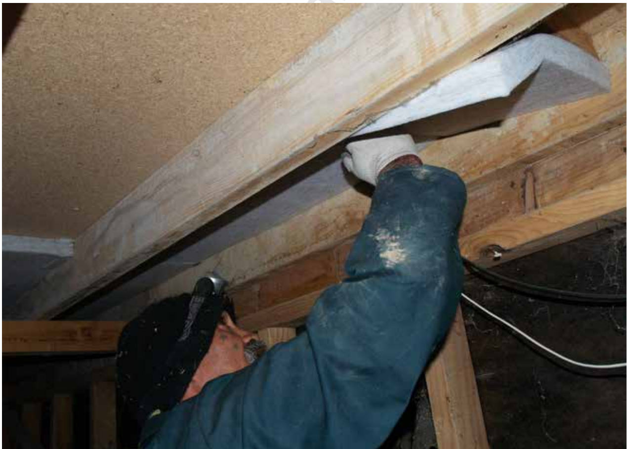
Figure 32 – Fitting semi-rigid sheets
