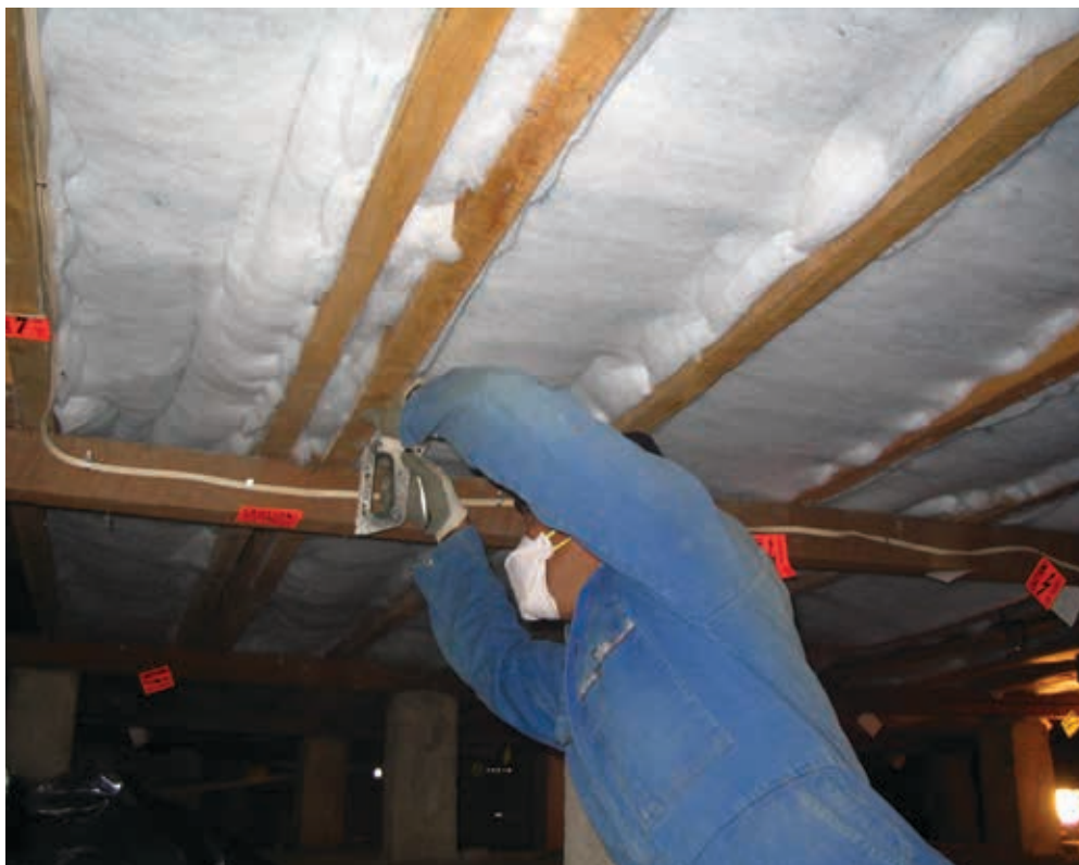
Figure 30 – Installed underfloor blanket
