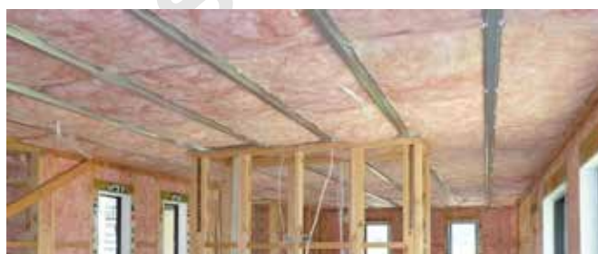
Figure 27 – Segments installed in a ceiling
